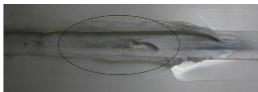
Figure 4.13. External voids and deformations on the weld surface, adapted from [59].
