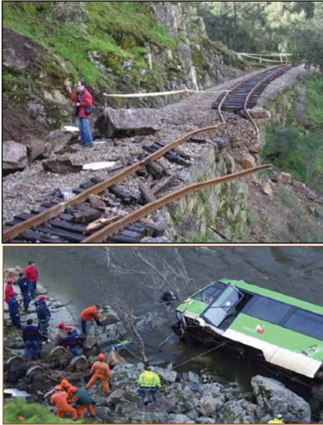
Figure 4. Complex slope movement affecting a railway near Carrazeda de Ansiães (February 2007).
