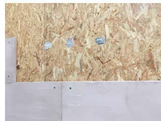
(a) PCM gypsum board over OSB panels.
