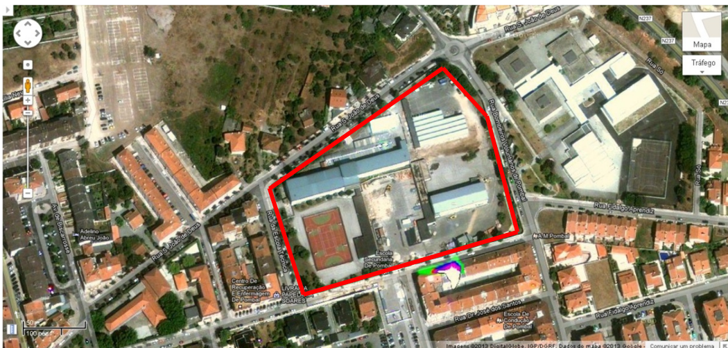
Figure 20 – Escola Secundária de Pombal | Aerial view (pre-intervention)
