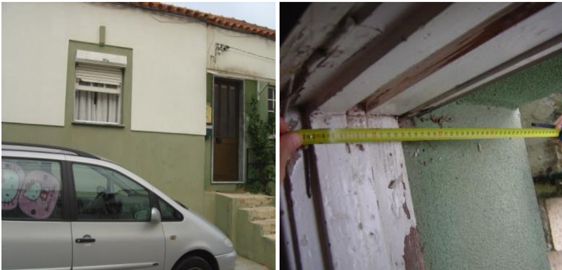
Figure 3-1 The case study: view of the single-family house
